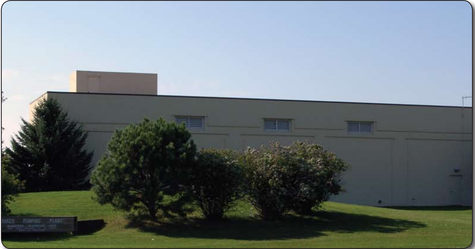
A 1.25-mile earthen canal conveys water from the James River to the Oakes Pumping Plant (pictured), where it is lifted 27 feet into the Oakes Canal.
