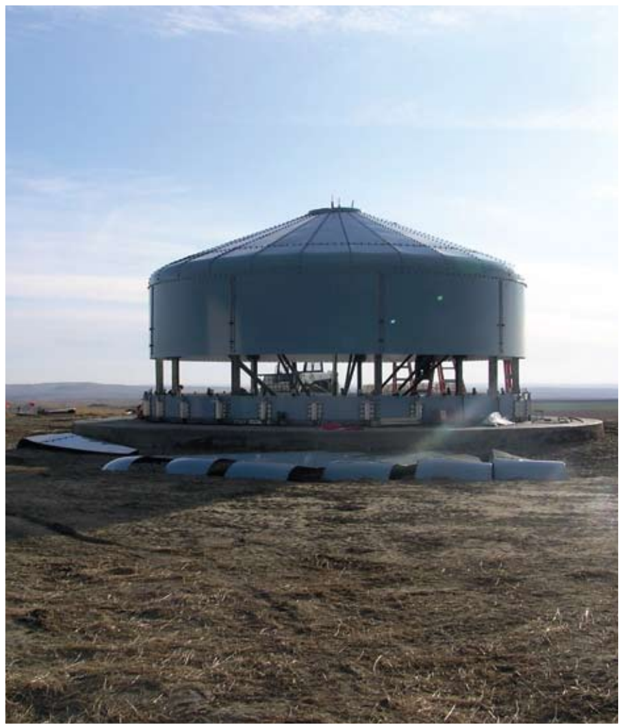
An off-site water storage tank for South Central Regional Water District was constructed with stimulus money.
