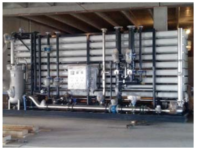
This photo shows the filtration equipment at the new SWPP water treatment plant.
