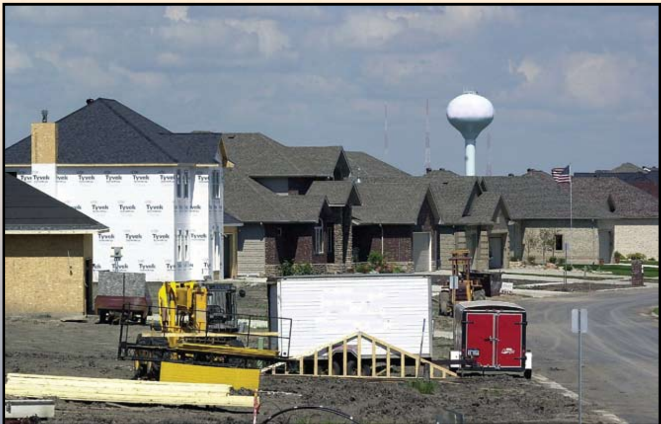
As the population of the Red River Valley grows, a supplemental water supply is essential. If a 1930s-type drought would occur today, it would take 1,200 truckloads of water per day, or one truckload of water arriving every minute around the clock for five months to supply the basic household water needs of Fargo alone.
