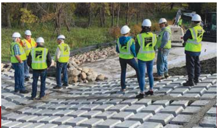
Garrison Diversion board members and staff learning about the construction of the discharge structure, located six miles south of Cooperstown near the Sheyenne River.
