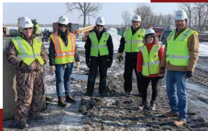
As construction was just getting underway, Garrison Diversion staff and directors visited the Missouri River intake site, located 4 miles south of Washburn.
