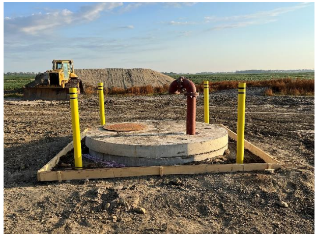
Typical air release manhole
