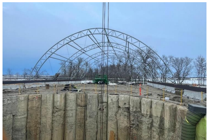
Winter Enclosure Structure
