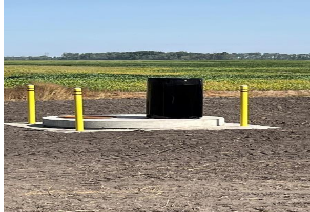
Typical Air Release Manhole
