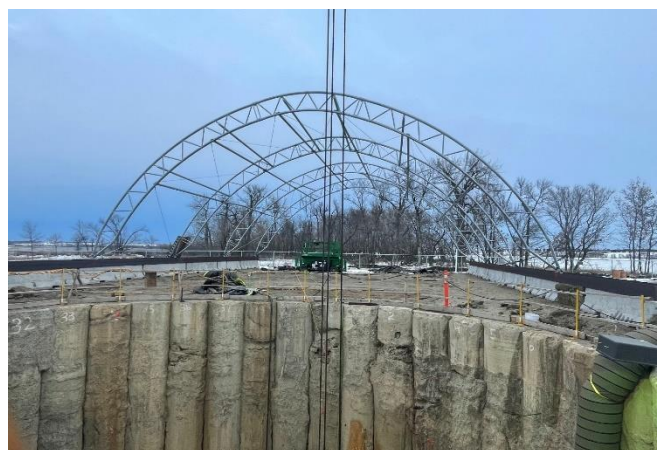
Winter Enclosure Structure
