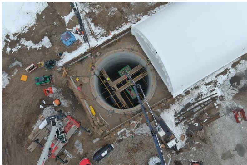
Concrete Pour on Divider Wall Inside the Wet Well
