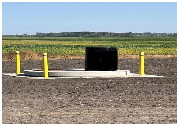
Typical Air Release Manhole
