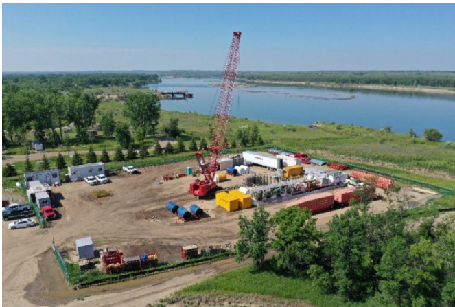
Site Under Construction
