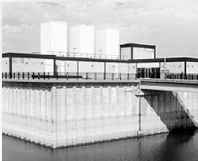
Snake Creek Pumping Plant
