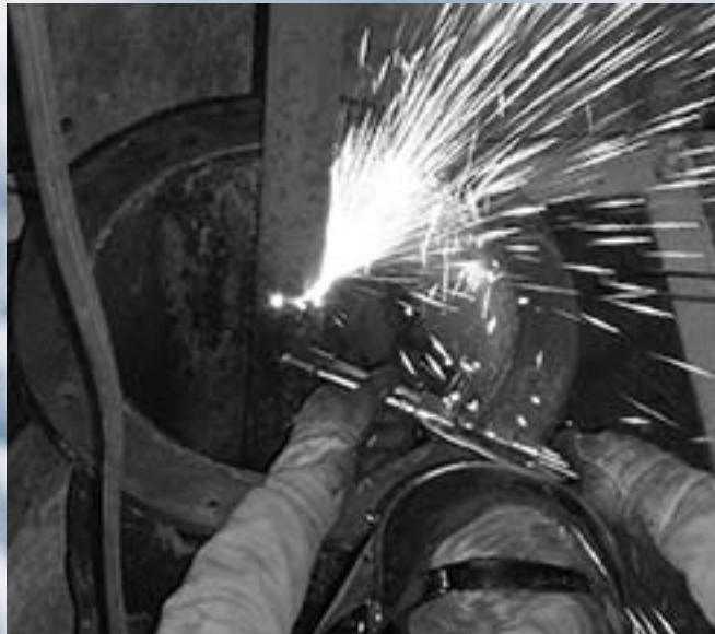
O&M workers refurbishing pump at Oakes Pumping Plant
