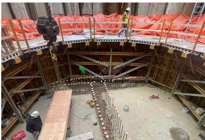
Liner Work on Rebar & Concrete Forms
