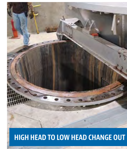
SCPP TUNNEL #2 MAINTENANCE
