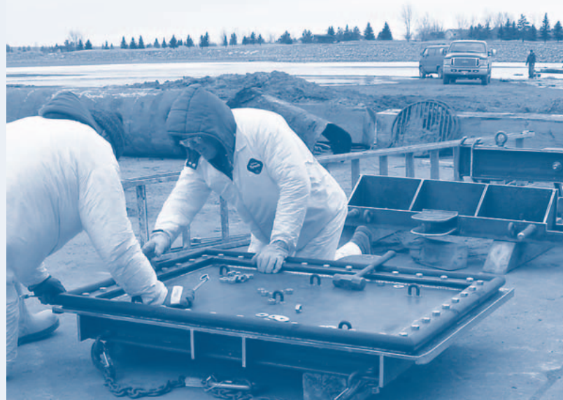
O&M workers performing maintenance activities at Dickinson Dam
