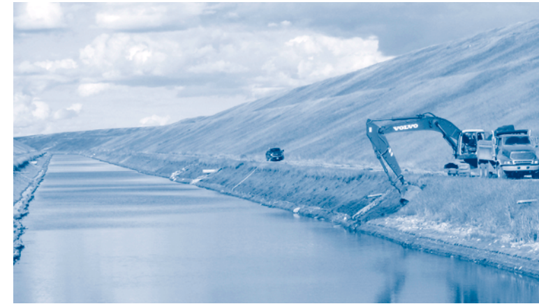
Slope-shaping at the McClusky Canal.
