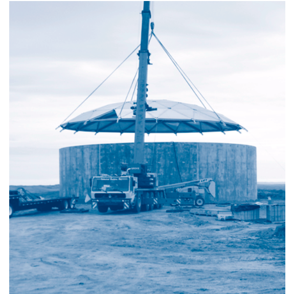
South Central Regional Water project.
