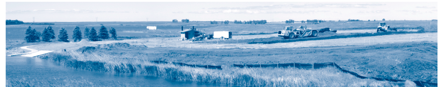
New John's Lake north boat landing construction.
