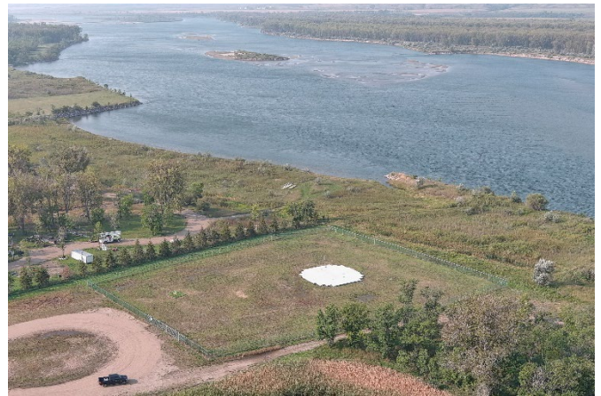
Completed Missouri River Intake
