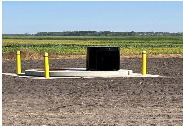
Typical Air Release Manhole
