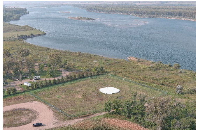
Completed Missouri River Intake
