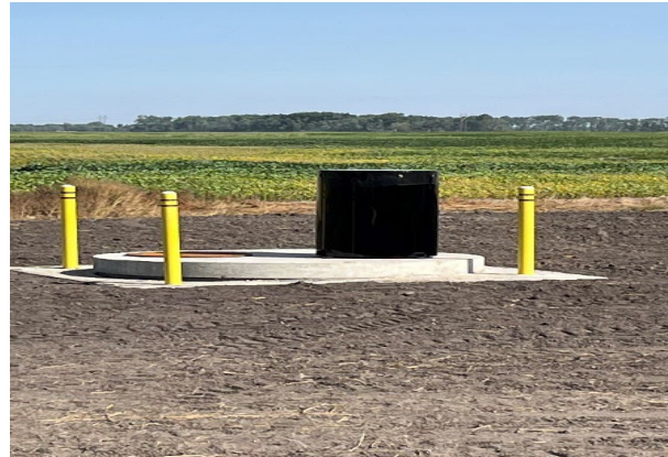
Typical Air Release Manhole
